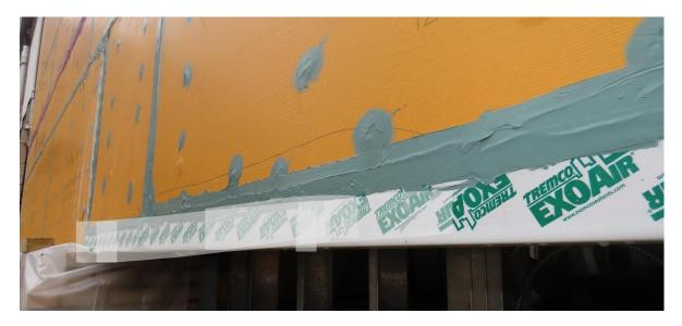
Air Barrier Flashing Detailing (1.0 hours, 1.0-AIA HSW)
